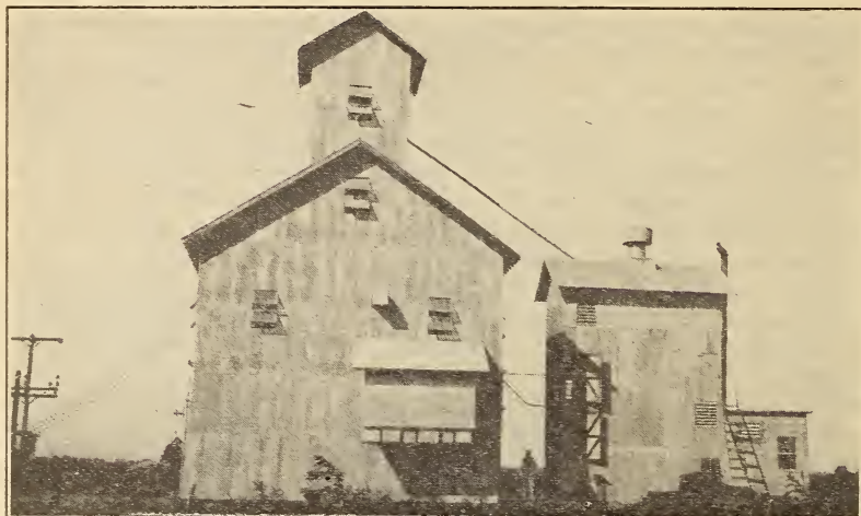
FIGURE 6.—Elevator and drier installation on a farm near DeWitt, Ark.
